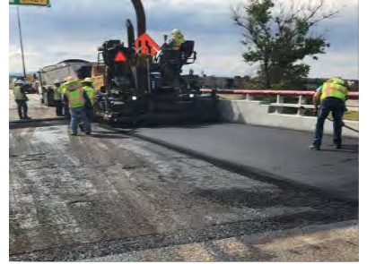
Image: Pavement overlay on the roadway
