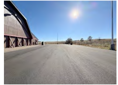
Image: Pavement at MSS-E
