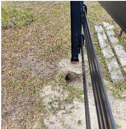
Figure 2-16 – Prairie Dog tunnel at snow fence post foundation
