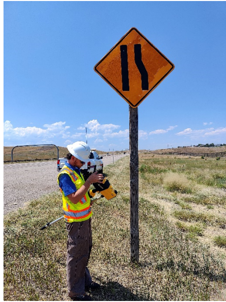
Figure 2-13 – Faded peeling sign near TPE
